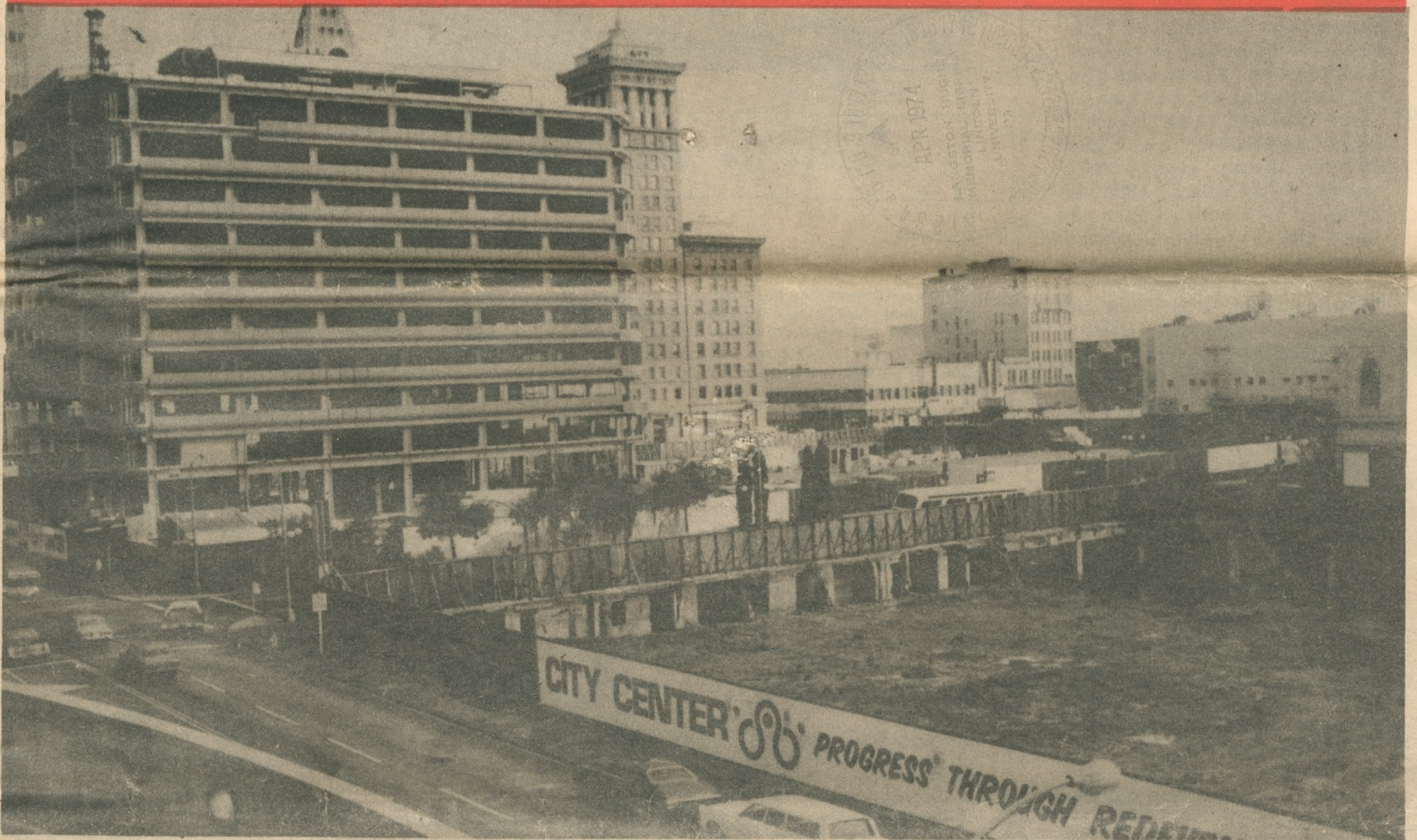
City Center Project construction sites.
